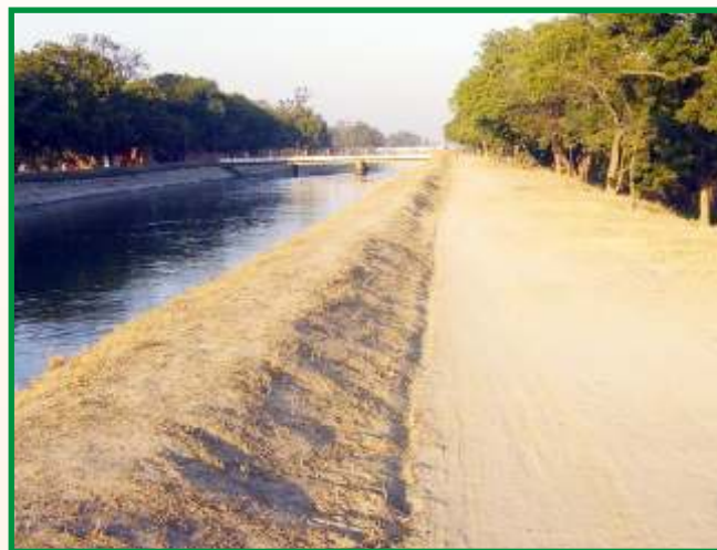
Plate 4. Canal embankments could be developed as water- front parks
