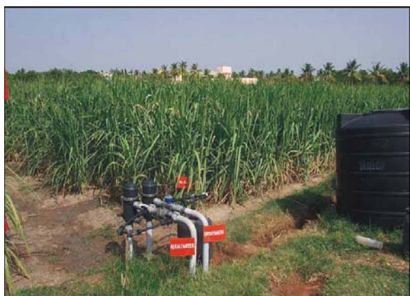
Distillery Spent Wash Treatment for alkali water using drip irrigation.
